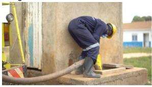
Figure 6: Safe Emptying of a lined toilet
