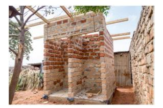
Figure 7: Lined facility under construction
